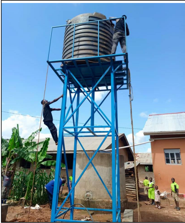
Figure 5: Installation of the Gentex 5,000 litre plastic tank.
