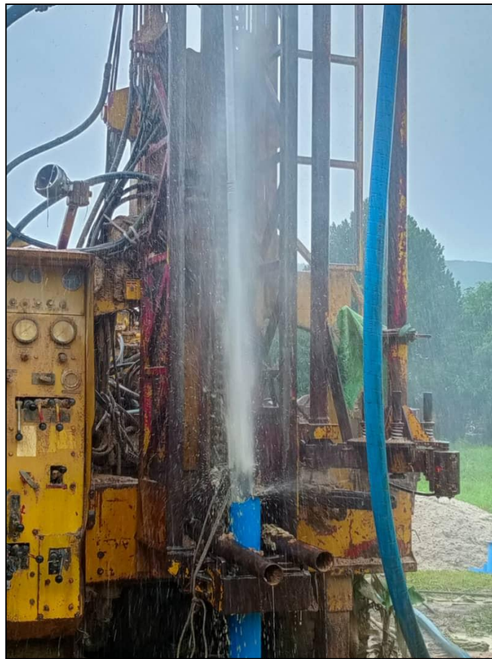
Figure 2: Borehole development
