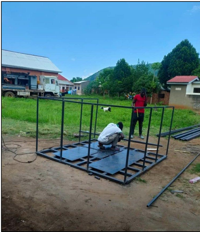
Figure 4: Construction of the steel tank stand
