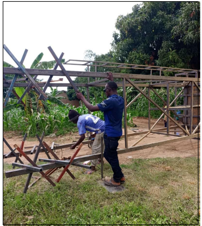
Figure 4: Construction of the steel tank stand
